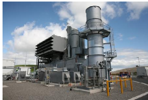
Electricity generation using modern peaker technologies
