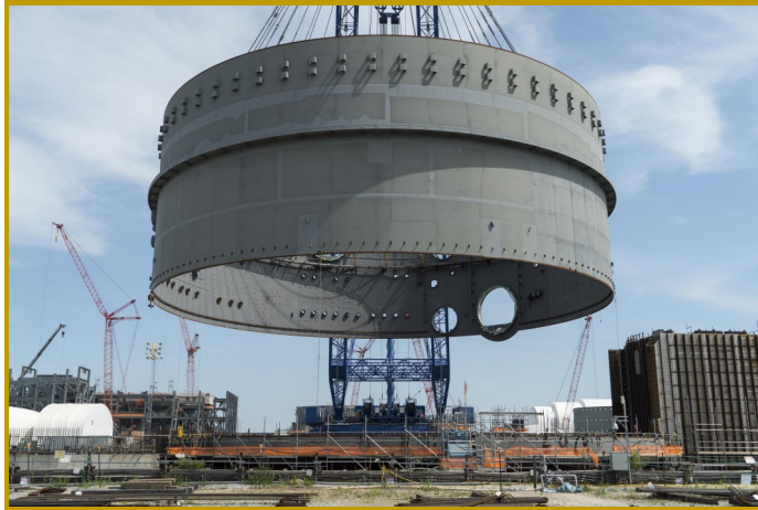
Containment rings are set at the Summer project in South Carolina.
