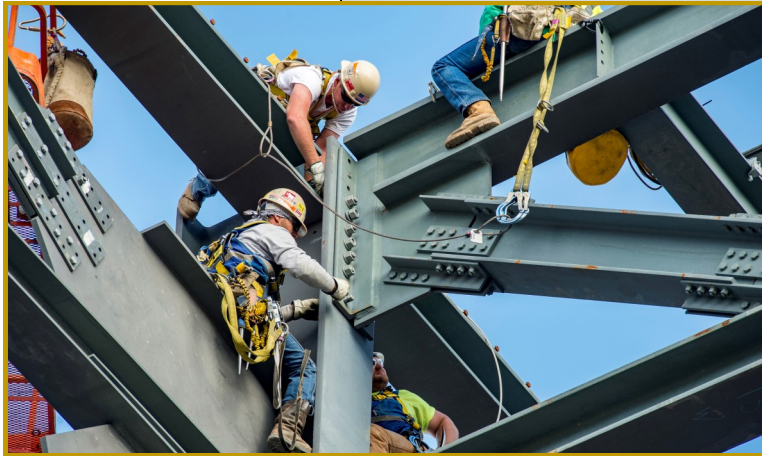
Workers set the final roof truss for the Vogtle Unit 3 turbine building. Photo: Courtesy of Georgia Power Co.
