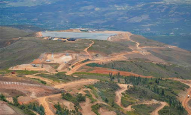
Shahuindo is Tahoe Resources' second gold operation in Peru and is already processing 10,000 mt/d. Photo courtesy of STRACON GyM.
