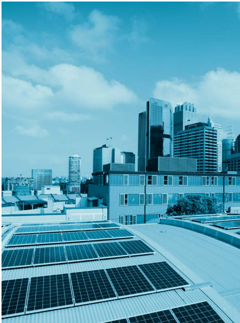
Rooftop solar panels, Sydney Australia Source: Shutterstock
